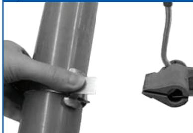
Remove tool, holding stub of band down with thumb.
